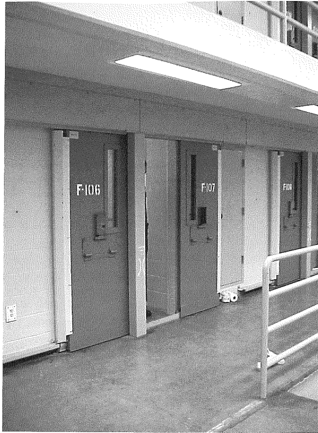
Figure 1. Control unit tiers. From the perspective of someone facing the cells, the doors that seal the pods are to the left and right and the control booth is to the rear. Photo by Allan R. Adams.
